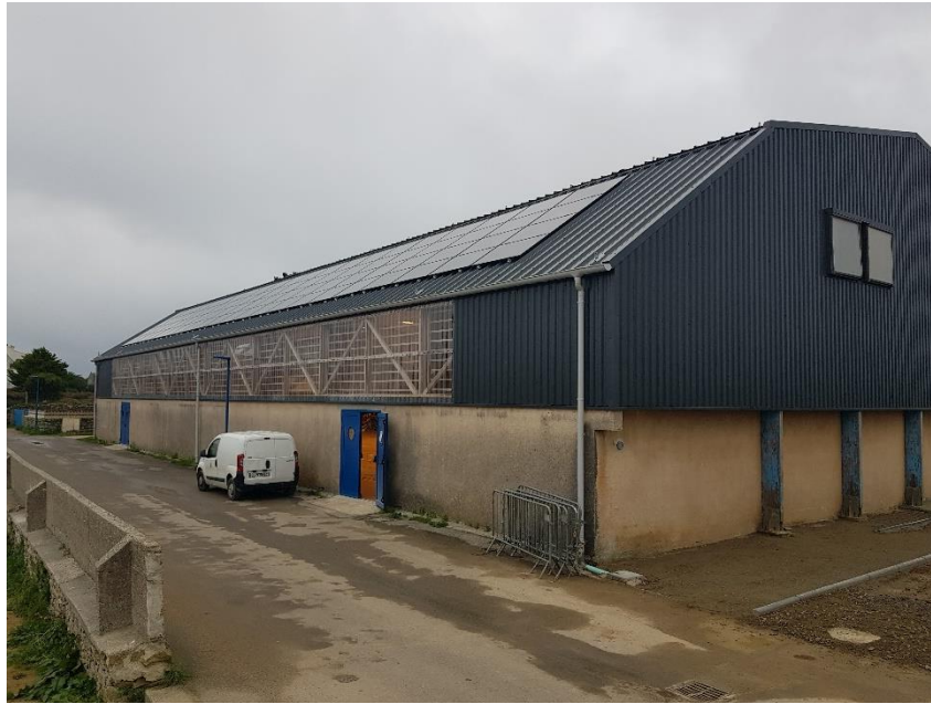
Figure 2.13 The sports centre building on Ushant showing the lower half of PV installation.
