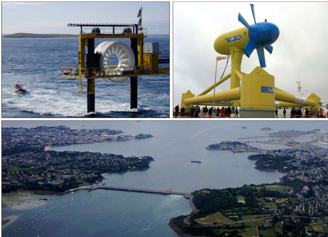
Figure 3-3: Examples of tidal power technology: OpenHydro turbine deployed at EMEC (Source: OpenHydro, 2018) (top left); Sabella D10 turbine (Source: Open Ocean, 2015) (top right); La Rance tidal power plant (bottom).
