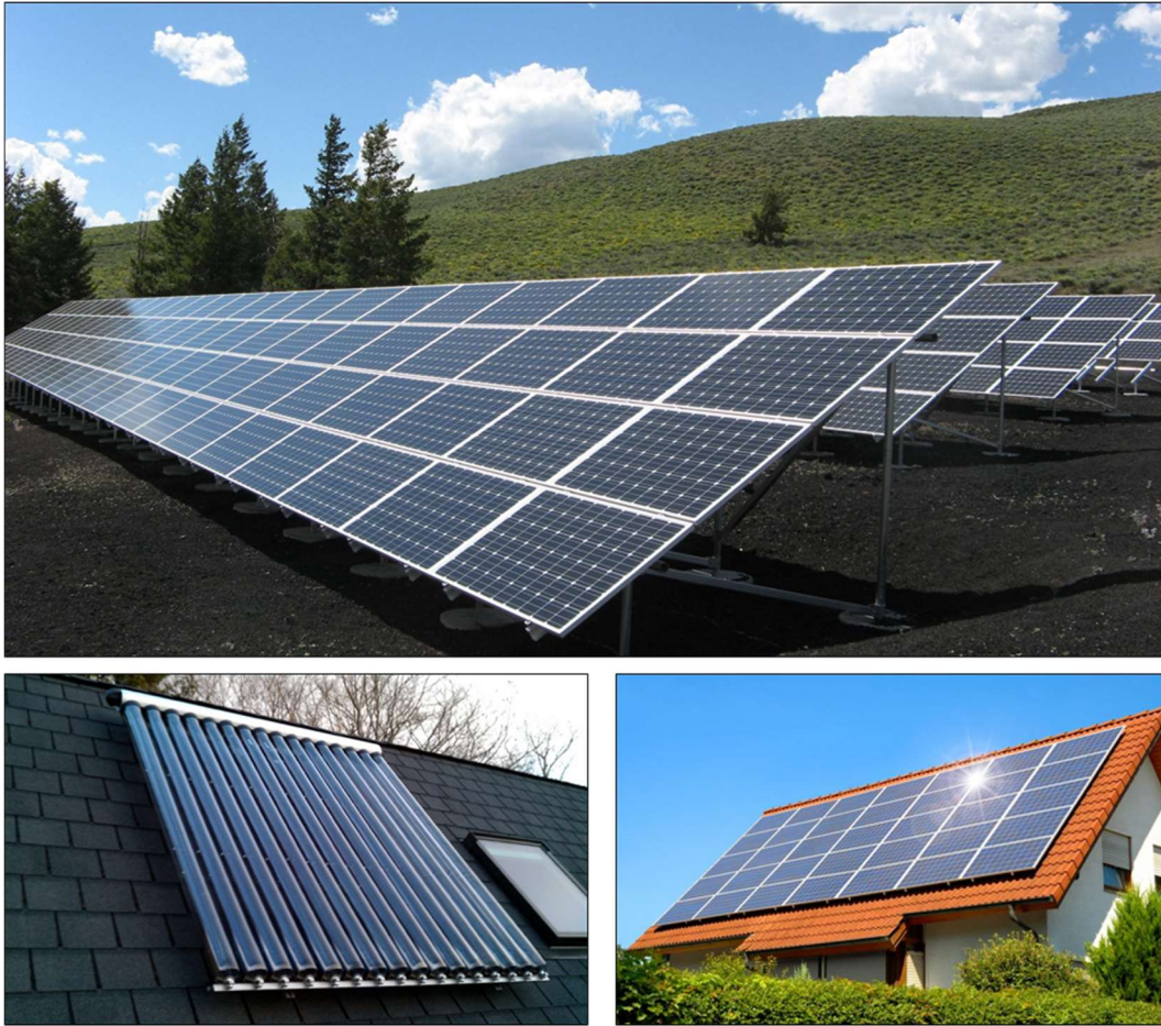
Figure 3-1: Examples of solar energy installations: ground mounted PV installation (top); rooftop mounted solar thermal (bottom left); rooftop mounted PV (bottom right).
